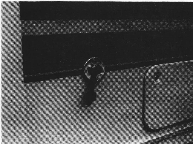
City Water Hook Up
